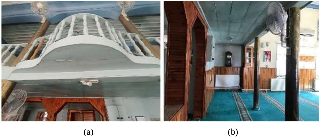
Figure 5.a. Protrusion of mahfil, b. Mahfil lower ceiling covering
