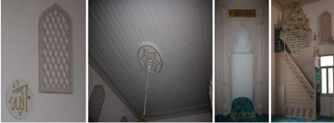
Figure 10.a. Upper Windows, b. Ceiling of the Harim, c. Half-Circular Profile Niche and Quarter Sphere Arched Mihrab, d. Wooden Pulpit 38
