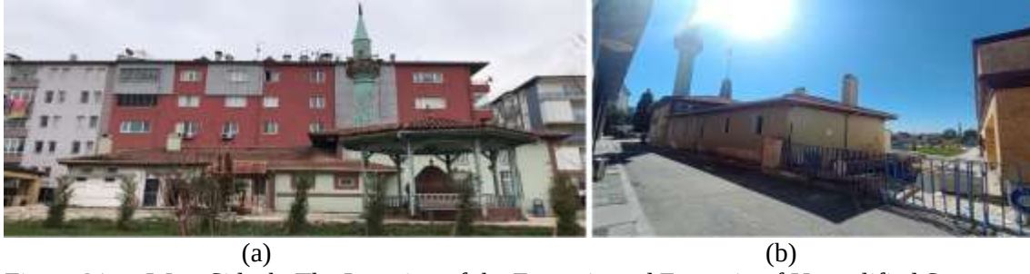
Figure 21. a. West Side, b. The Location of the Fountain and Fountain of Unqualified Structures Joined from the North Side (2024)
