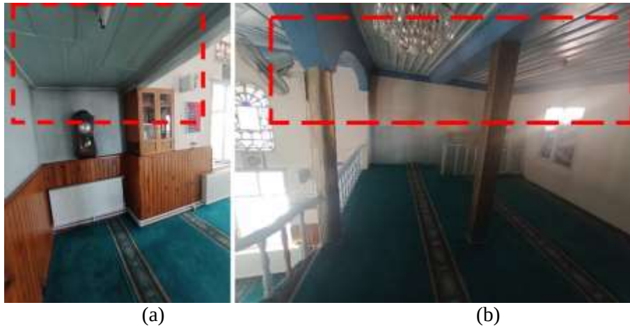
Figure 17.a. Trace of the Closed Exit of the Gathering Stairs on the Gathering Ceiling Covering, b. Lathed Ceilings of the Gathering and Last Congregation Place on the Gathering Floor.
