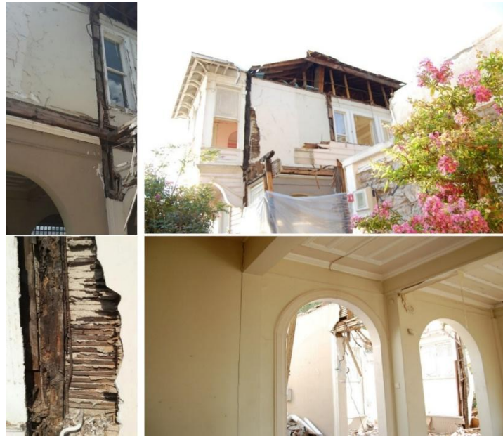
Figure 2. Rotten Wood Prop, Baghdadi Cement Over Lath, Pembe Yalı Interior, Damage Caused by Reinforced Concrete and Steel Columns Added to the Structure for Strengthening (Author, 2017).
