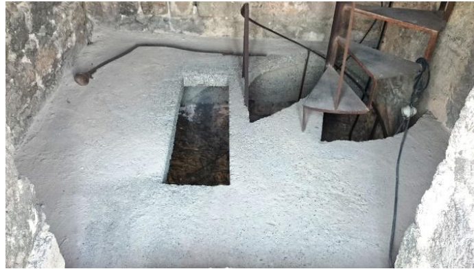
Figure 8. Reinforced concrete slabs and iron staircase.
