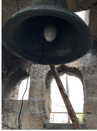
Figure 9. One of the bells with a lamp is mounted on the reinforced concrete slab in the clock pavillion section. 36
