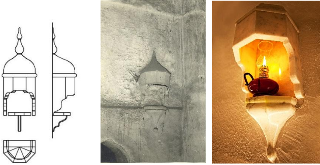
Image 21. Drawings of the Çerağman made on archival photographs and a photograph of the space before and after the application, 2020.
