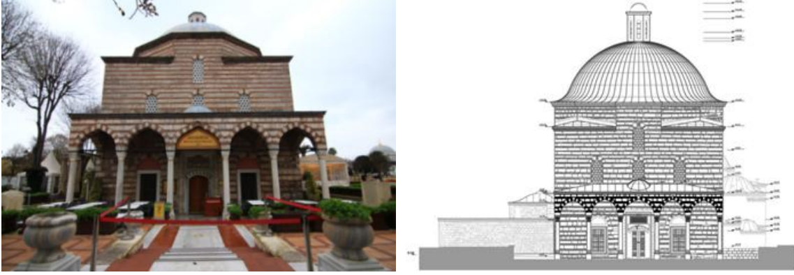
Image 6. Photograph of the men's entrance door of the bathhouse in December 2020 and a survey drawing of the entrance façade (author's archive).
