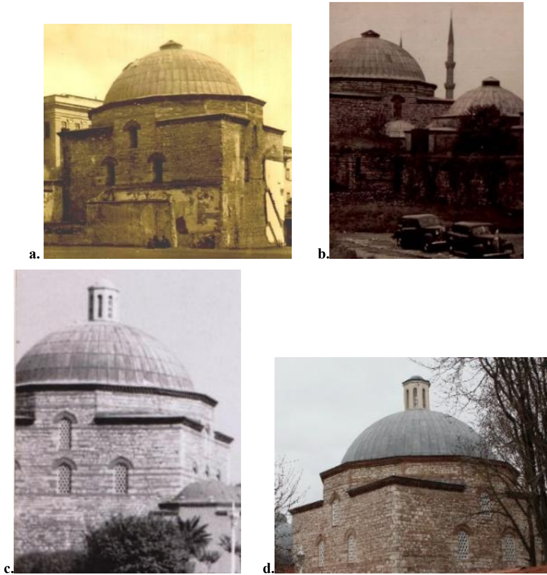
Image 14. Photographs showing the status of the light towers on the cold room domes in a. 1942, b. 1978, c. 1986, and d. 2010, respectively (author's archive).
