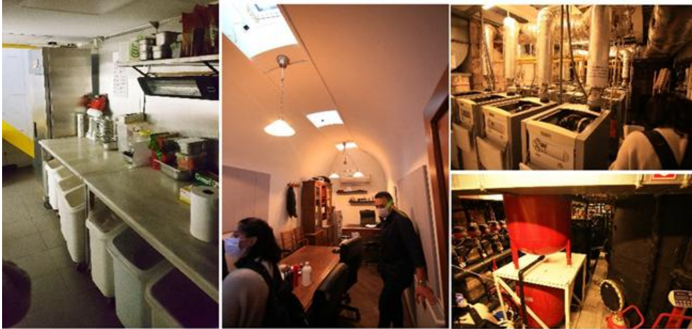
Image 23. During the re-functionalizing of the building, the upper level of the furnace, which was turned into two floors by taking advantage of its height, was converted into a kitchen area, the lower level into a plumbing room, and the cold water tank into an office area(author archive).
