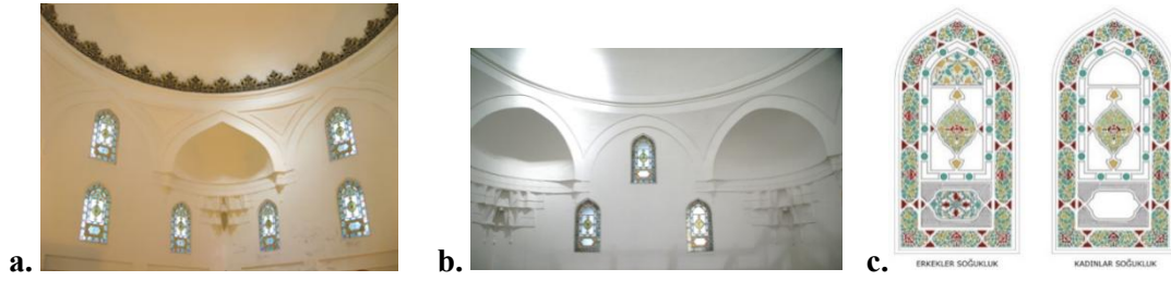
Image 12. Photographs from 2010, when the changing rooms in the cold section, which is accepted as a 1986 addition, were dismantled during the restoration. In the pictures where the revzen windows, dome decorations, and muqarnas can be observed comparatively, the one on the left (a) belongs to the men's cold room and the one on the right (b) to the women's cold room, c. In the drawings made for the revzens in the cold sections during the survey studies, it is seen that there are fewer embroidered applications in the women's section compared to the men's section (author archive).
