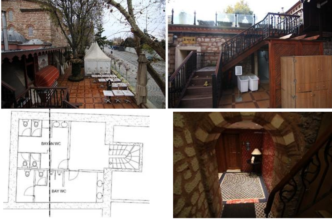
Image 23. The additions made to the facade of the building to provide the expected comfort level and service variety in the restaurant services provided by the business prevent the perception of the facade and the integrity of the building. Survey drawings of the restrooms built with a new project on the lower elevation of the furnace and a photograph of the entrance to the space (2021).
