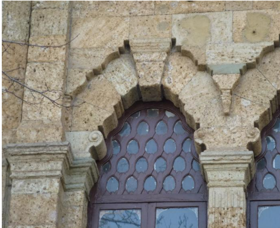
Photo 12. Detail of 1 st Floor Windows' Arches and fluted column of the Janissary Museum (Kuleli, 2015)
