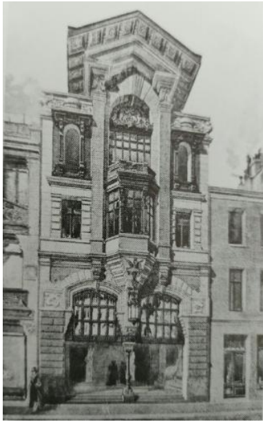
Figure 11. A House Project Known as House with Small Columns 1896. (Barillari and Godoli, İstanbul 1900 Art Nouveau Mimarisi ve İç Mekânları , 61)
