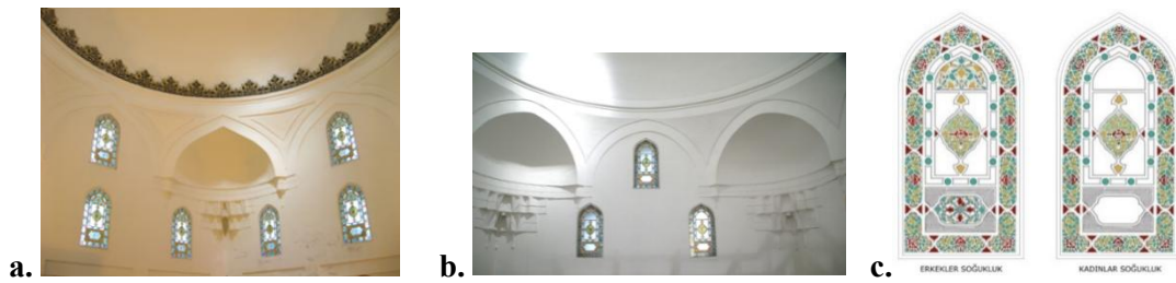
Image 12. Photographs from 2010, when the changing rooms in the cold section, which is accepted as a 1986 addition, were dismantled during the restoration. In the pictures where the revzen windows, dome decorations, and muqarnas can be observed comparatively, the one on the left (a) belongs to the men's cold room and the one on the right (b) to the women's cold room, c. In the drawings made for the revzens in the cold sections during the survey studies, it is seen that there are fewer embroidered applications in the women's section compared to the men's section (author archive).
